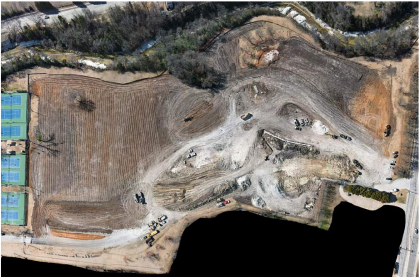
Rick Oden Park Construction Aerial Photo, courtesy of Bobby Hensley
